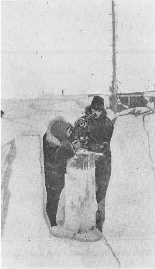
FIG. 3. Taking transit observations during the first winter at Collinson Point, Alaska. Conducting such scientific observations in the cold taxed the men and equipment. Source: Chipman and Cox, "Geographical Notes" (ref. 30), 44B.
